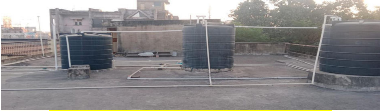
Boring Storage capacity: Water tank of 5000 L Capacity
